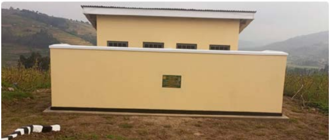
Newly constructed 3stance VIP latrines at hamurwa primary school Rubanda district
